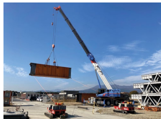
A device for guiding suspended loads with ropes "EG-Guide"
