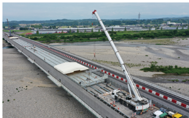
Hokuriku Expressway Tonami Interchange to Kosugi Interchange deck replacement work
