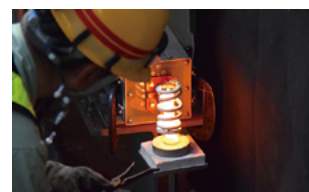
New method: By rapidly heating the rivets with a heating coil and shortening the distance to the installation site, there is no longer a need to throw high-temperature rivets, which improves both work efficiency and safety.
