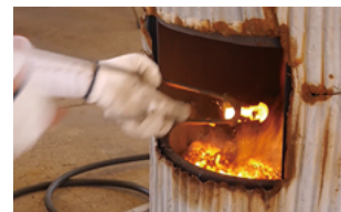
Traditional method: Required skilled work such as throwing high-temperature rivets heated by coke to workers
