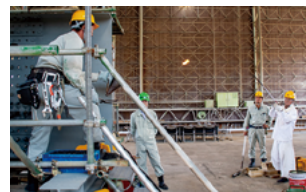
Traditional method: Required skilled work such as throwing high-temperature rivets heated by coke to workers
