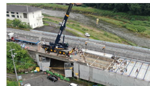
Deck replacement work using KK Rationalized Joints, a proprietary jointing method
