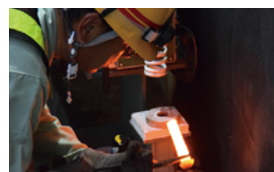
New method: By rapidly heating the rivets with a heating coil and shortening the distance to the installation site, there is no longer a need to throw high-temperature rivets, which improves both work efficiency and safety.
