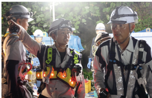
Removing the Sugitani No. 2 Overpass
