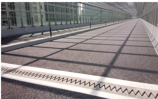
KMA Joint on the Kachidoki Flyover
