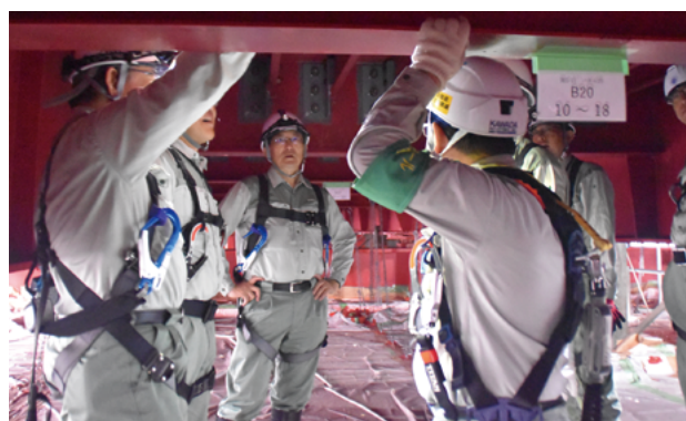
Patrolling the narrow space at a bridge construction site
