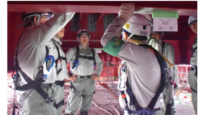
Patrolling the narrow space at a bridge construction site
