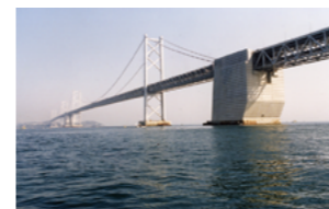
Minami Bisan-Seto Bridge (1988, Kagawa Prefecture)
