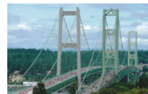
New Tacoma Narrows Bridge (2007, Washington State, US)
