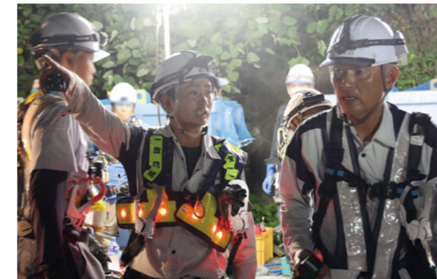
Removing the Sugitani No. 2 Overpass
