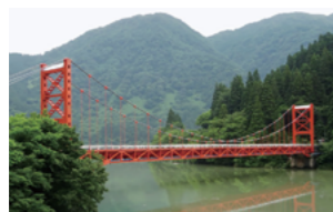
Owatari Bridge (1958, Toyama Prefecture)
