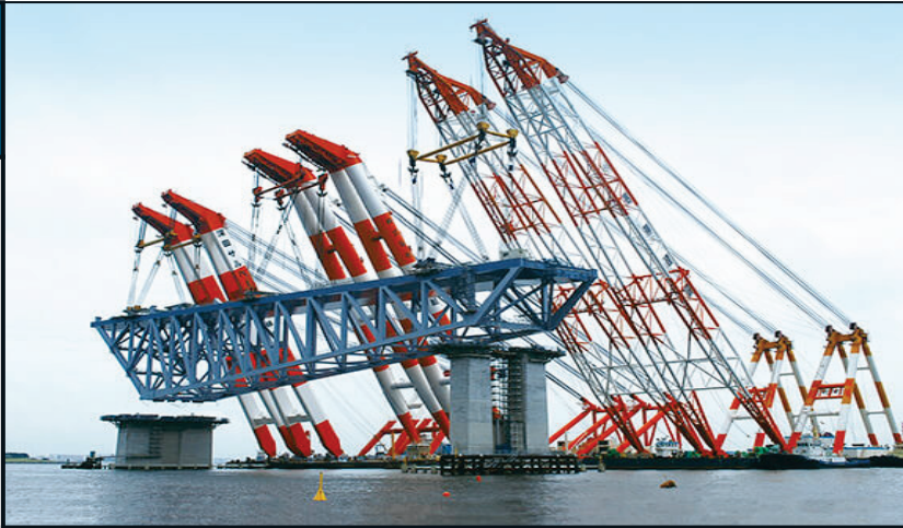
Tokyo Gate Bridge (Tokyo)
